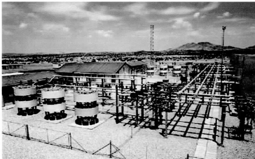
Figure 2.1 : 1 Auas static var compensator
