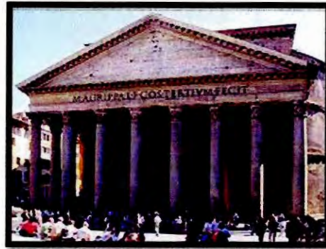
Figure 2.1: Hadrian's Pantheon in Rome is an example of Roman concrete construction.
