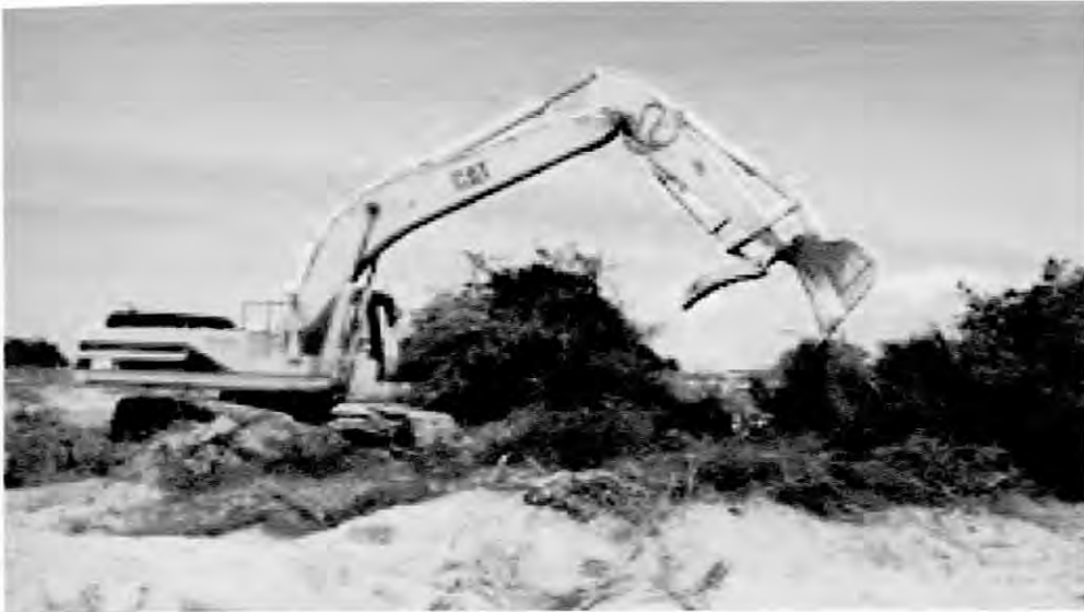
Figure 2.4b. A large backhoe on an excavator.
