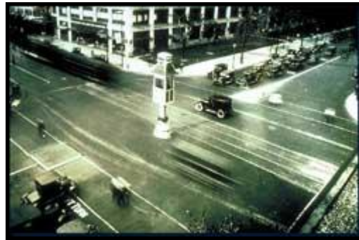
Figure 2.2: Traffic tower (Regenold, 2007)
