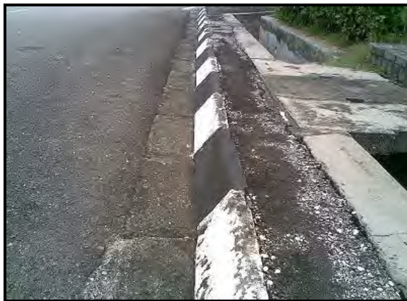
Figure 1.2: Road side curb after painting
