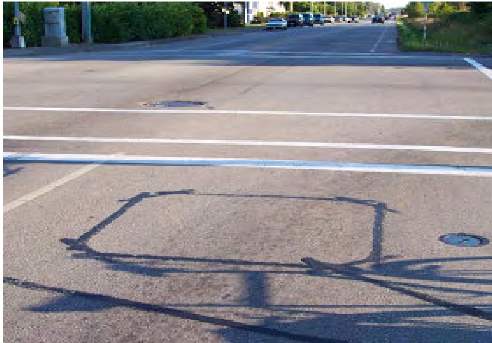
Figure 1.3: Sensor mounted on the surface of road in traffic light
