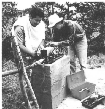
Figure 2.2: A Colombian manufacturer (right) installs a DC Pico-hydro Generation System
