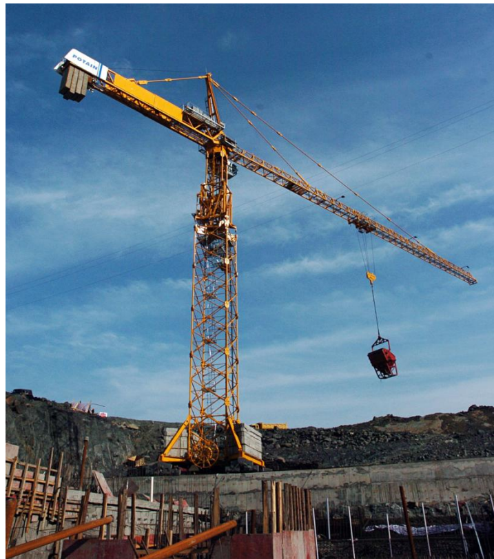
Figure 2.3 Rotary or Tower Crane
