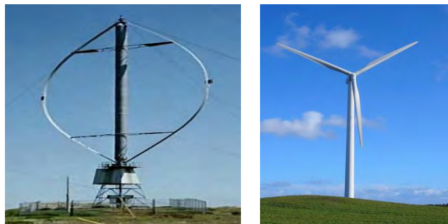
Figure 2.4: Vertical (left) and horizontal (right) wind turbine
