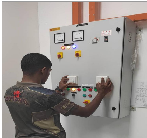
Figure 3.15 Chamber Thermostat Setting
