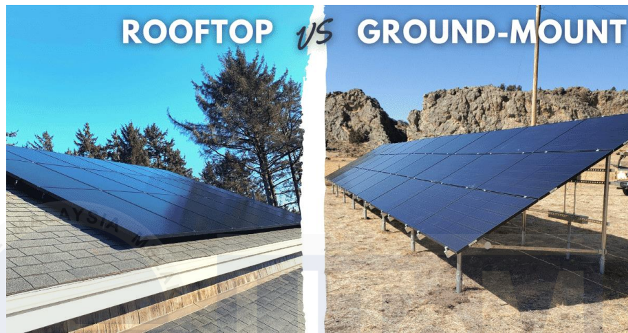
Figure 2.7 Example of Roof-mounted structure compare to Ground-mounted structure that uses in Solar PV System [16]
