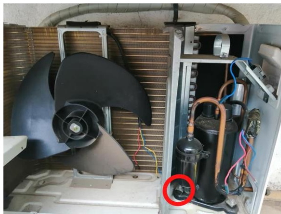
Figure 1.1 Location of rubber mounting in split unit air conditioning
