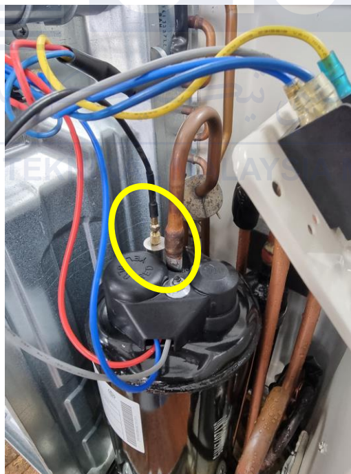
Figure 4.3 Vibration sensor at the top of compressor (near to copper pipe)
