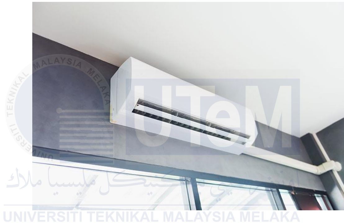
Figure 3.9 Example of Split Unit of a resident with NEM system
