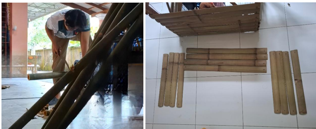
Figure 3.7 Bamboo cutting and installation process
