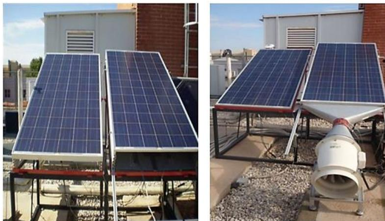
Figure 2.7 PV panel with air cooling and without air cooling [5]
