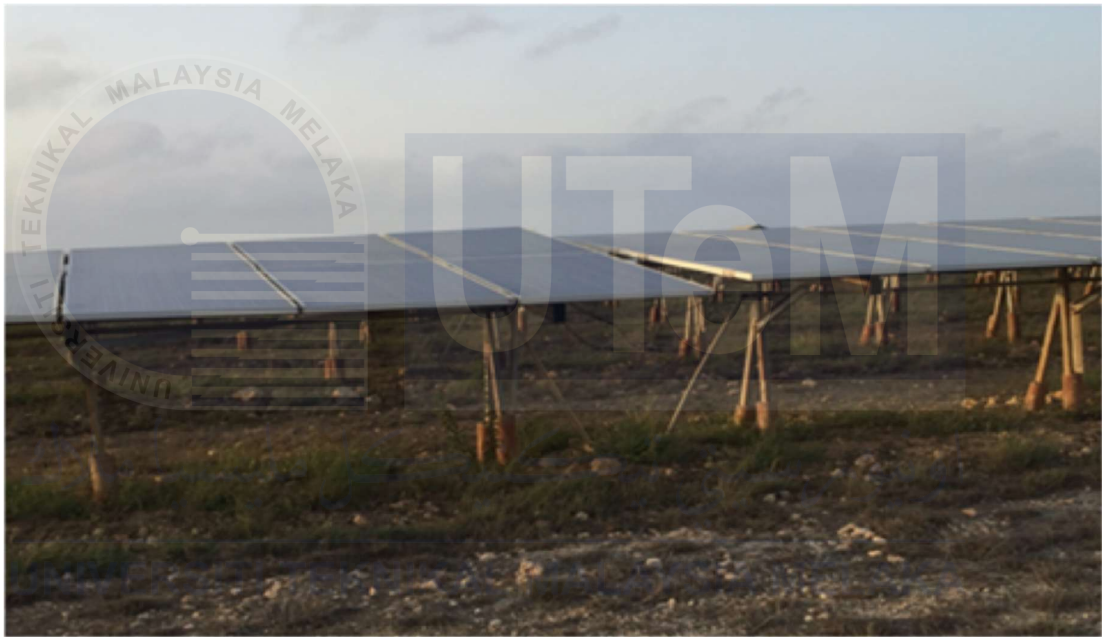
Figure 2.10 Uneven tilt for the adjacent solar arrays[15]
