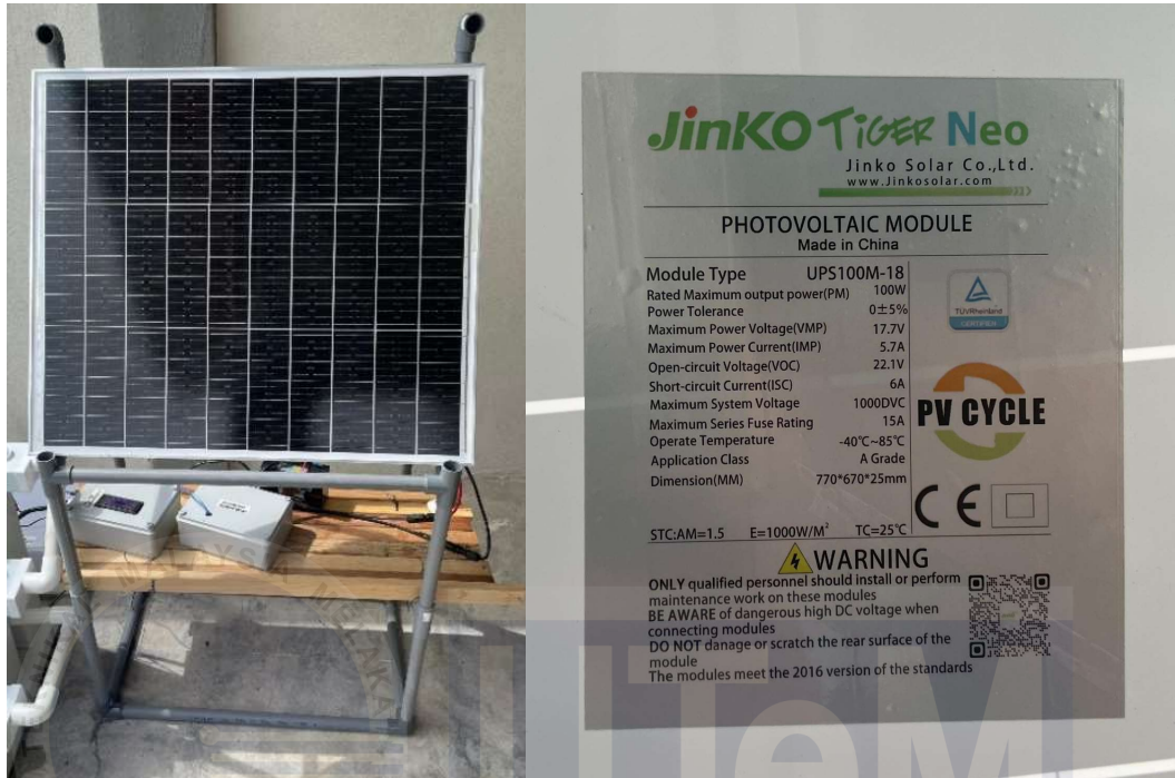
Figure 4.13 Solar Panel Placement
