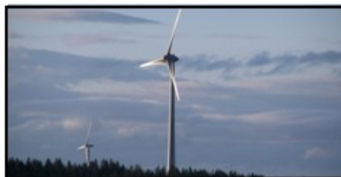
Figure 2.1 – Horizontal axis wind turbines
