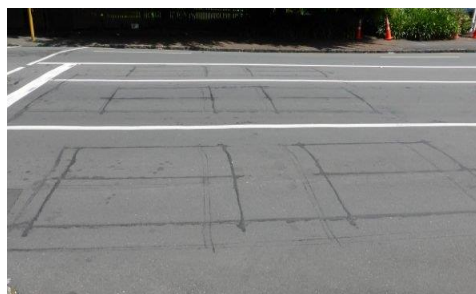
Figure 2.9: Induction Loop Buried in The Roadway
