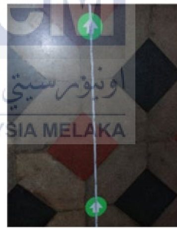
Figure 2.9 (b): Adhesion of PLM directional arrows on floor
