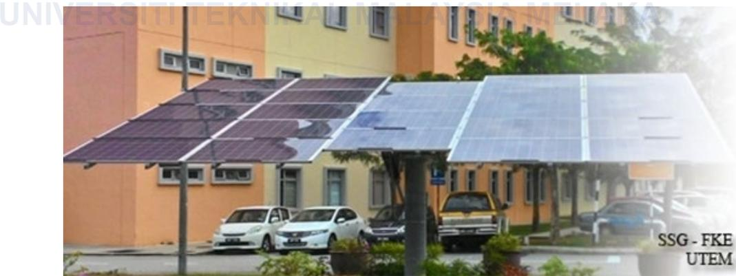
Figure 1.5: Polycrystalline solar panel at the FTKE entrance [8]
