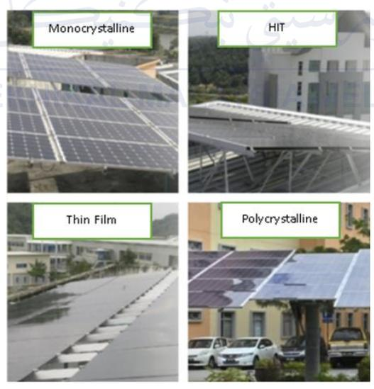
Figure 1.2: Types of solar panel at FTKE, UTeM [5].
