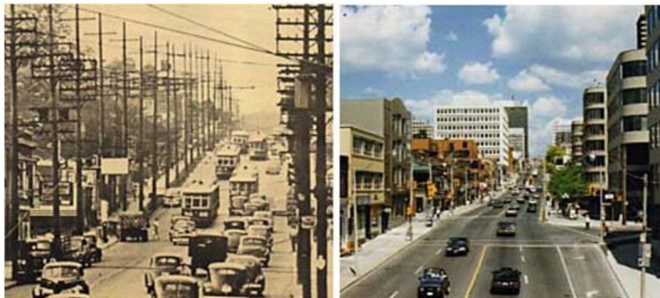
Figure 1.1 The difference between overhead and underground cable[1]
