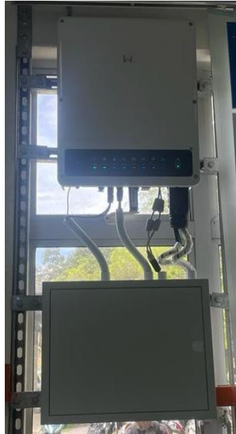
Figure 3.4: GoodWe GW5K-ET inverter
