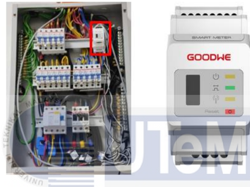
Figure 3.7: Smart Meter
