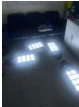
Figure 3.7 Lamp brightness inspection
