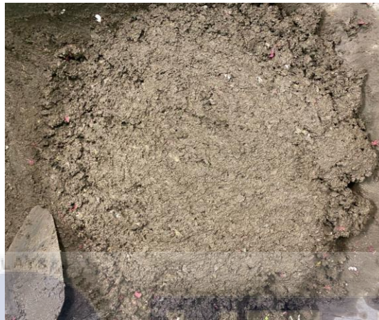
Figure 3.7: Uniform of concrete mixture
