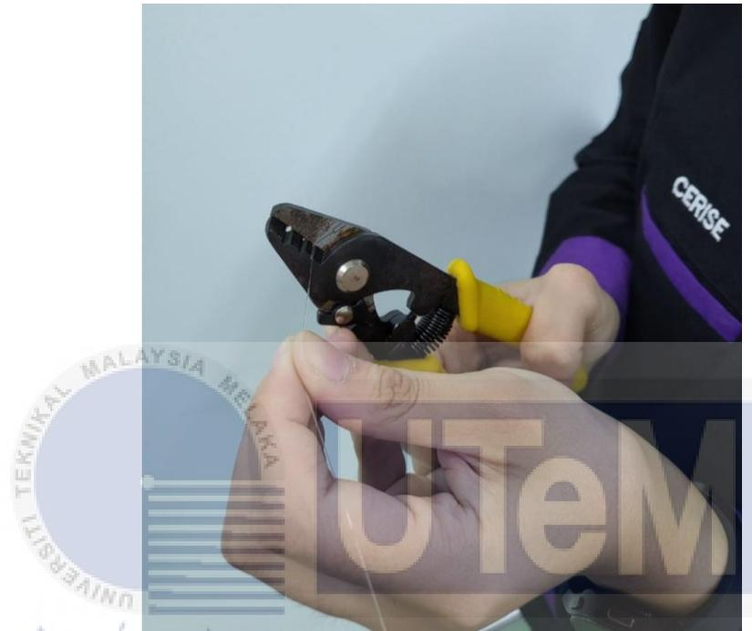
Figure 3.15: The process of stripping the fibre optic cable.
