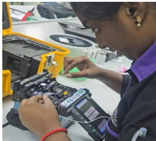
**Figure 3.14 : The process of splicing the fiber optic cable**
