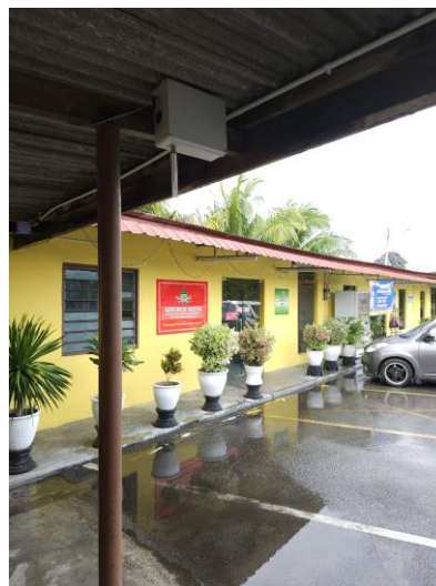
Figure 4.13: Gateway Located at Masjid Nur As-Sa'adah
