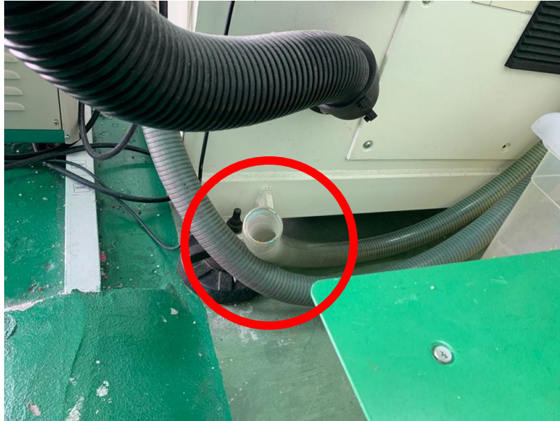
Figure 2.18 : Tube incompleted assemble
