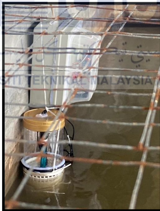
Figure 3.4: Mechanical setup for monitoring device.
