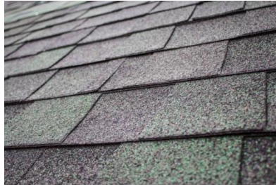
Figure 2.4: Asphalt shingle roof (Porter, 2020)
