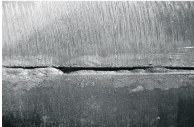
Figure 2.10: Lack of Fusion
