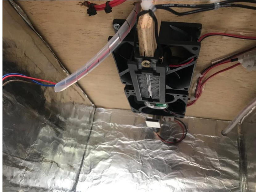
Figure 4.2 Fan and heater position inside box.
