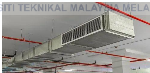
Figure 2.2: Air Duct Ventilation System
