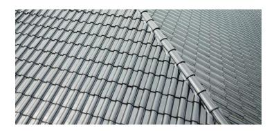
Figure 2.2 Clay roof tile
