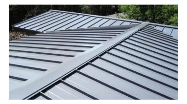
Figure 2.3 Metal deck roof
