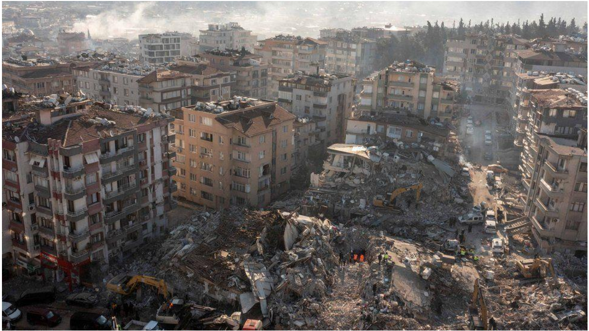
Figure 1.2: Damages done by the earthquake in Turkiye
