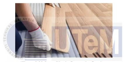
Figure 2.23 Stone Plastic Composite flooring
