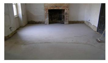
Figure 2.17 Concrete flooring
