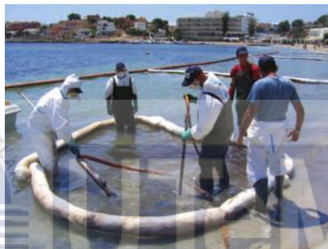
Figure 2.5: Adsorbent materials. (Source: Hammouda, 2021)
