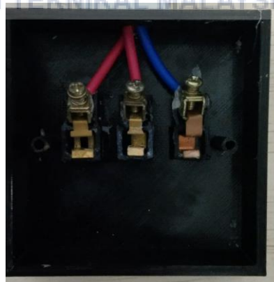
Figure 4.10 Wiring Base Installation
