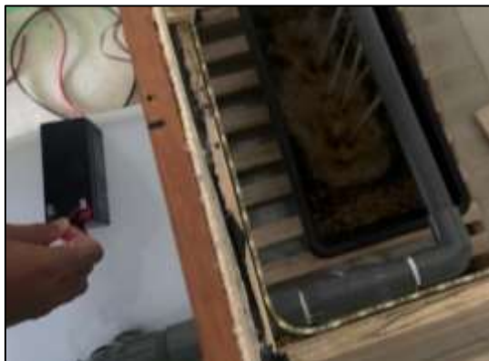
Figure 3.33 Test the Water Pump Pipeline
