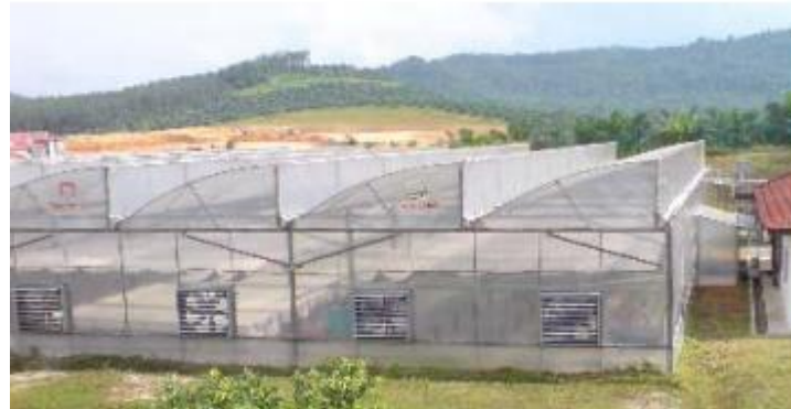
Figure 3 Four ventilation fans and planting channels inside the greenhouse.
