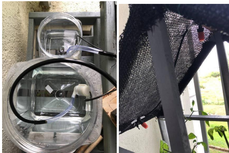
Figure 3.5 Irrigation and Fertilization System Pump Setup
