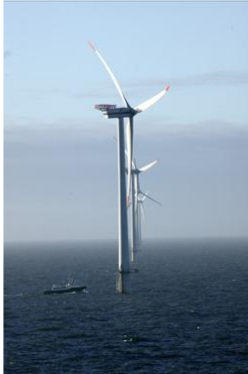
Figure 2.3 – wind generator in big scale.
