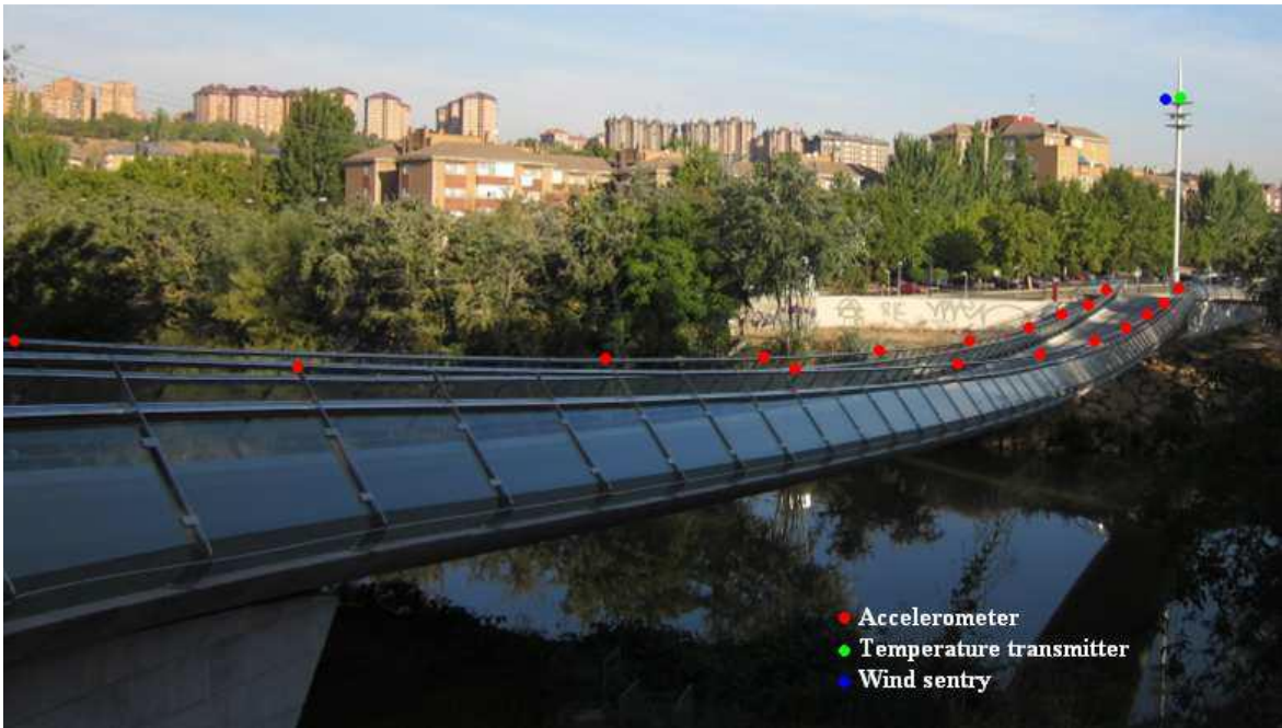
Figure 2.10 Structure bridge with aid of sensors distribution.
