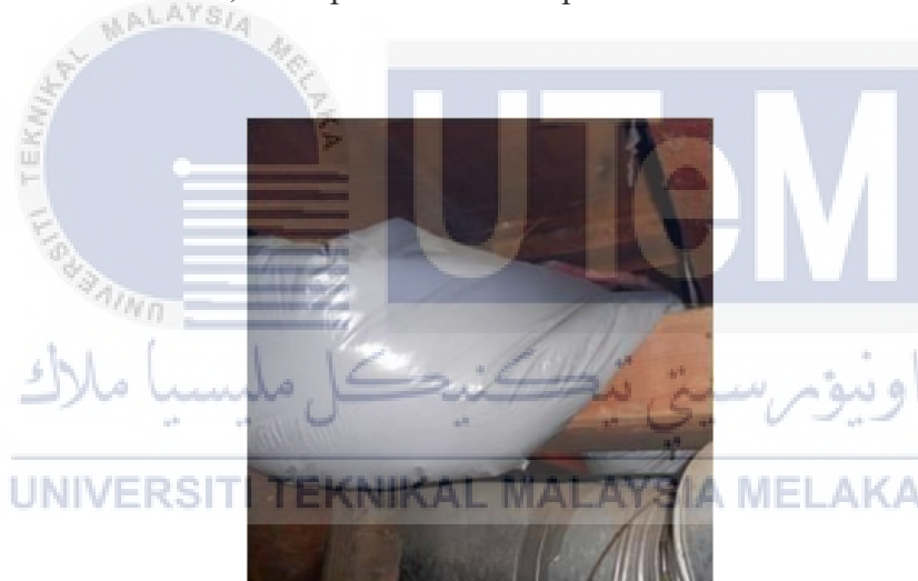
Figure 1.2. Flex duct comprises a plastic inner liner attached to a metal coil, a layer of fiberglass blanket insulation, and a plastic or foil vapor barrier.
