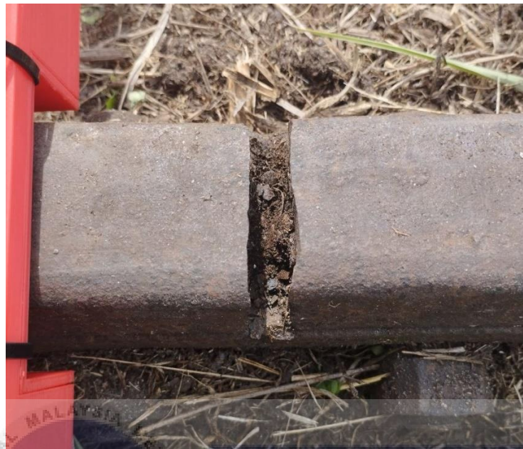
Figure 4.12: The crack at the railway
