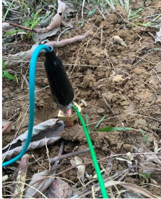
Figure 4.27 Copper Earth Clamp
