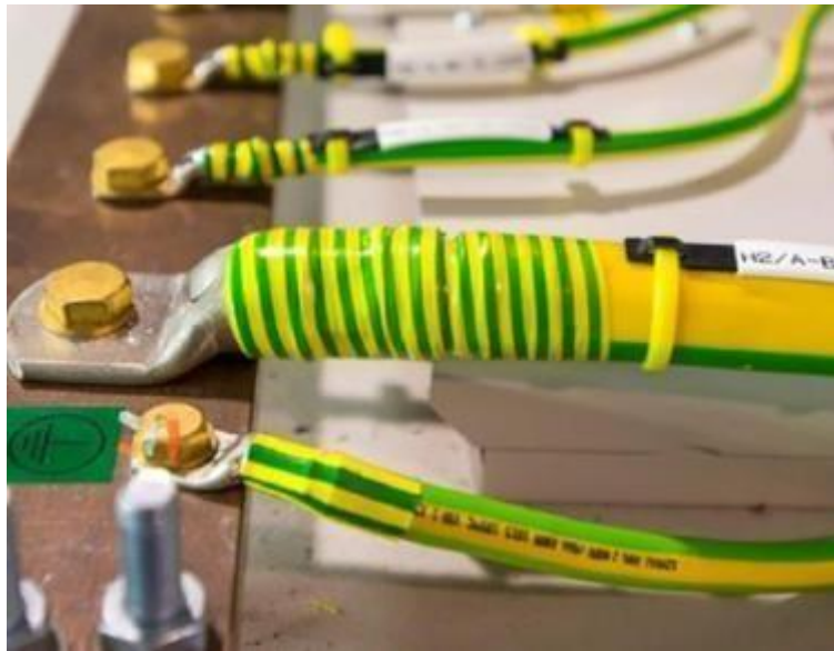
Figure 1.1 Electrical grounding wire [8]
