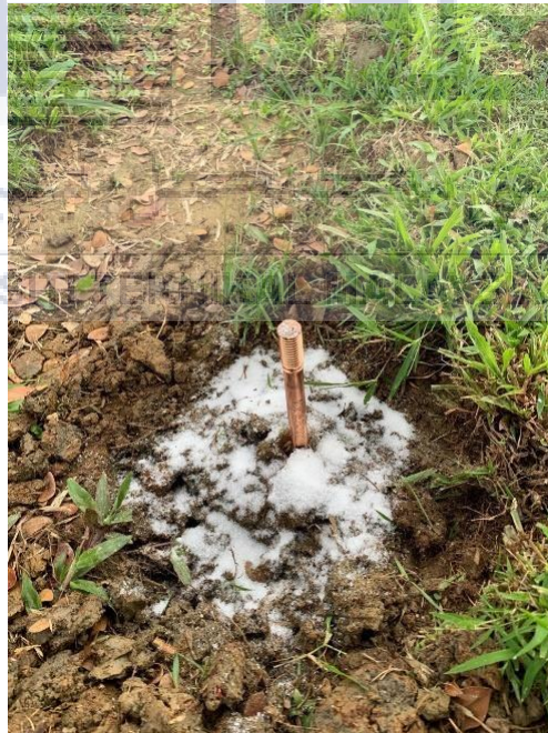
Figure 4.12 Epsom salt around electrode rod
