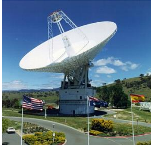
Figure 2 1 DSS-43 70-meter X-Band spacecraft communication antenna at Canberra Deep Space Communication Complex, Australia
