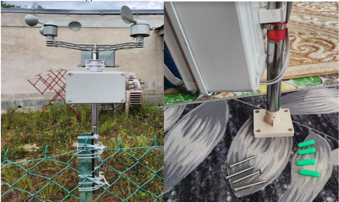
Appendix G Weather station installation method
